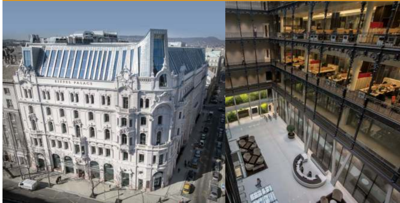
Projekt / Project: Eiffel Palace irodaház / Eiffel Palace Office Building
